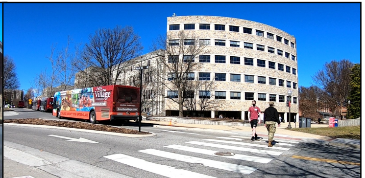
On the Virginia Tech campus, the crosswalk between Newman Library and Eggleston Hall, on a two-way street, was observed as part of the research project..
